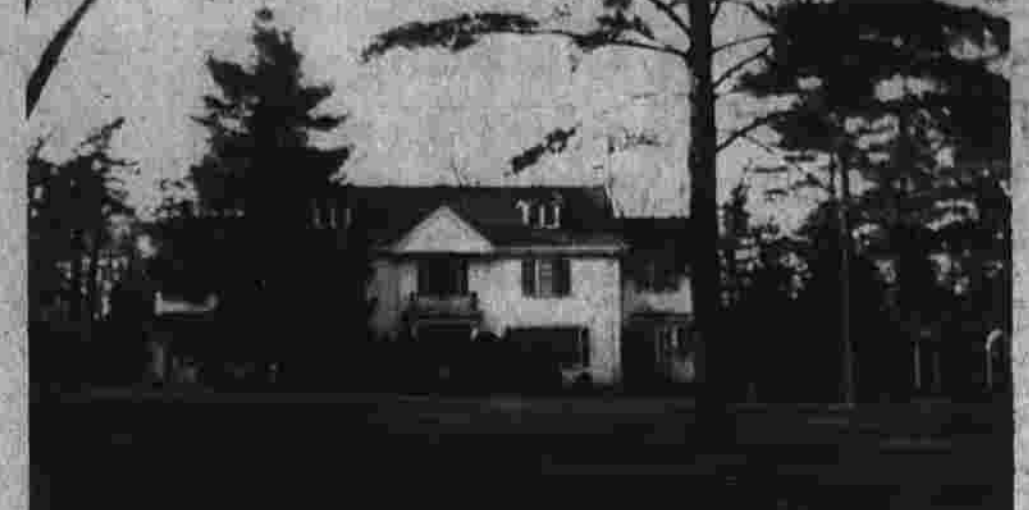
Littlewood, built for the Cheneys at Park and St. James Sts.
